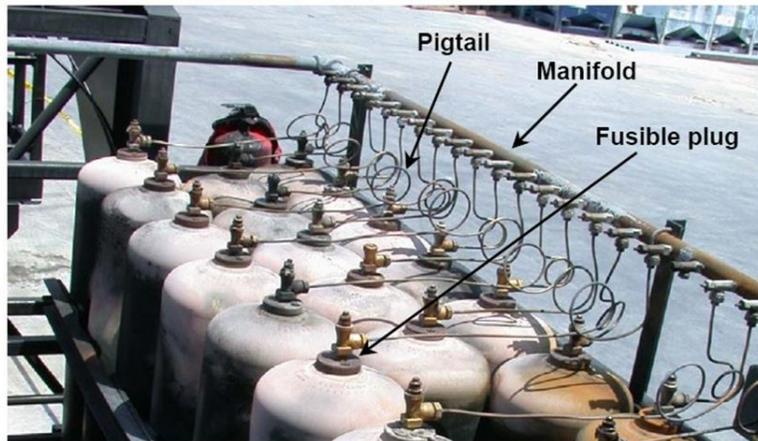
These have been involved in a number of significant facility or motor vehicle incidents. These must be approached with extreme caution as there can be multiple cylinder failures and fire. No effective method has been developed for these incidents other than flooding quantities of water from a distance to cool and prevent more cylinders from rupturing.
